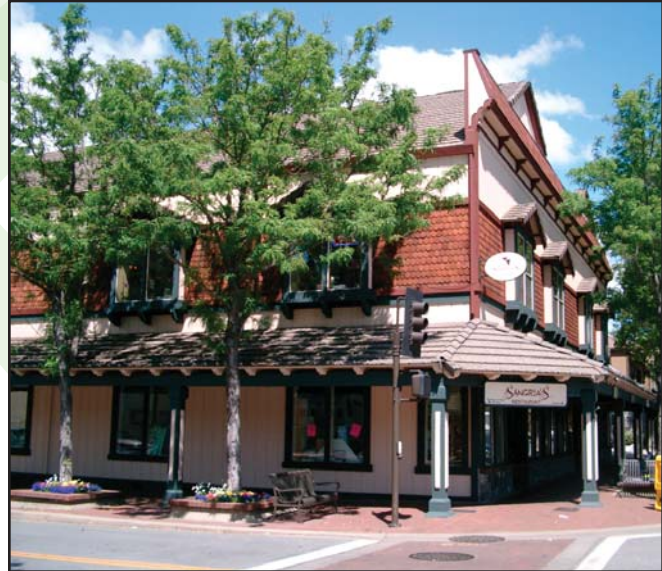
Pictured above is the Millhouse Mall Building. The new renovations are clearly seen on the second floor of the building creating a pleasant addition to Downtown.
